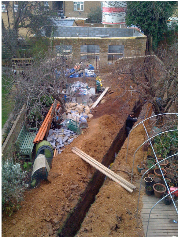
Drainage going in
